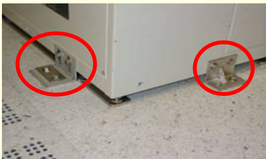
Diff: Furnace機台
