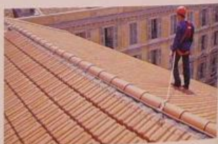
INSTALLATION ON ROOF RIDGE
